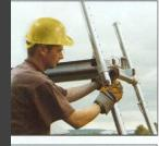
Release the support frame and swing out towards the eves of the roof. Engage the hooks so that the frame is angled towards the eves and not under the platform.
