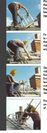
Place ridge unit over the ridge of the roof. Ensure that the wooden bearers are placed flat against the roof tiles.
